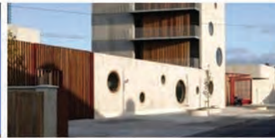
Sean o'casey centre, Dublin O'Donnell & Tuomey Architects
